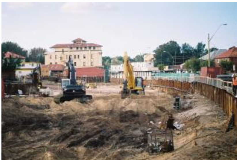
Figure 4: Basement excavation at Capella Apartments
