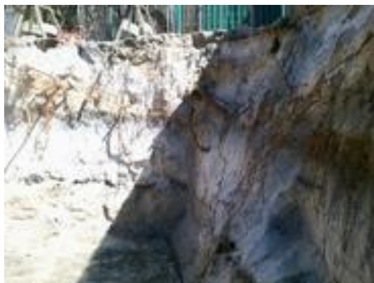
Figure 7: Grouted sand for 3m deep excavation at Minneapolis Crescent, Maroubra.
