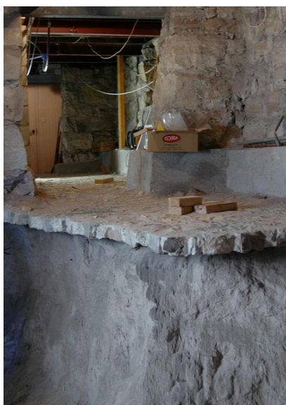
Figure 5: Grouted sand underpinning Beach Street, Coogee
