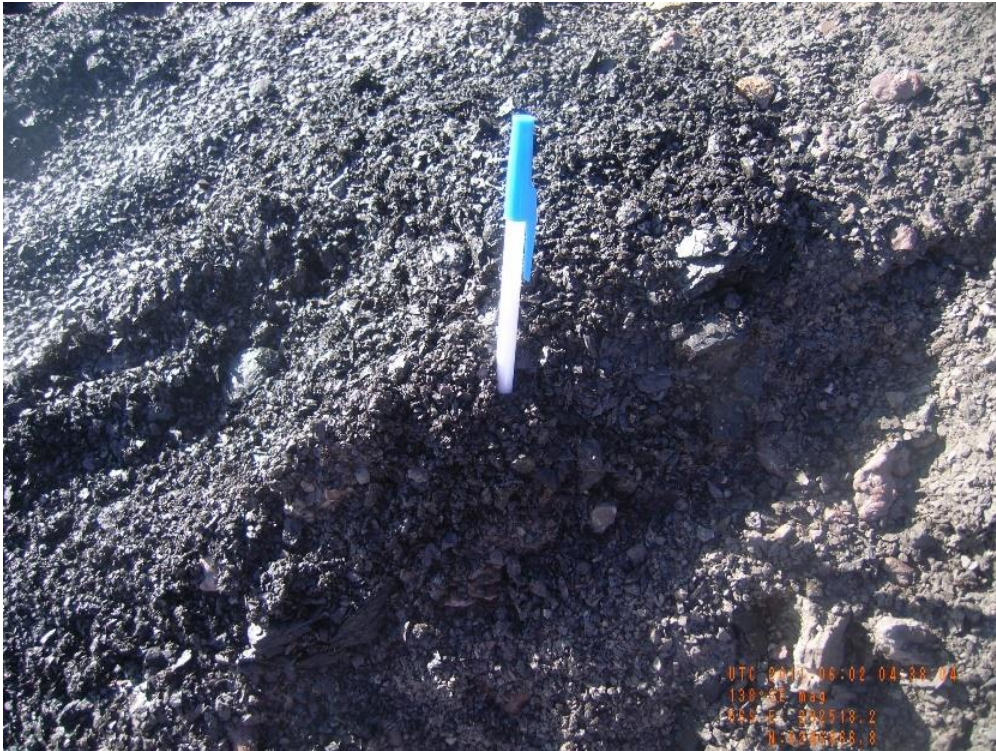
Figure 2: Observed degradation of Bringelly Shale
