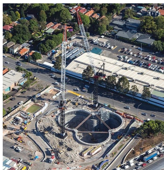
(b) Aerial image of shaft construction
