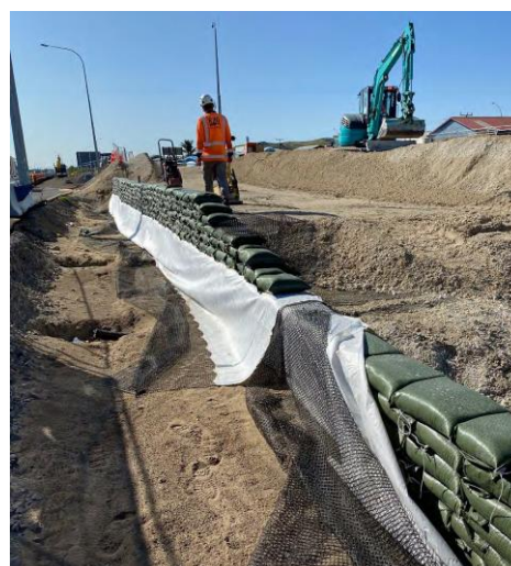
(b) Partially constructed MSE wall
