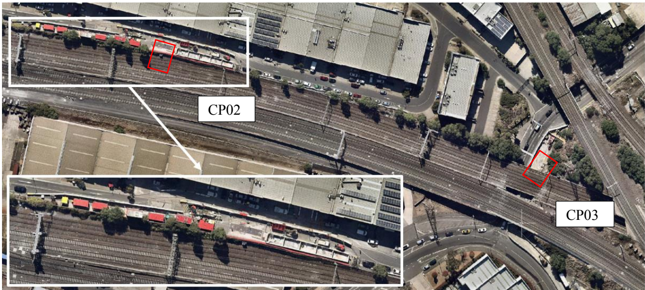
Figure 7: Site set up at Cross Passage CP02 and CP03
