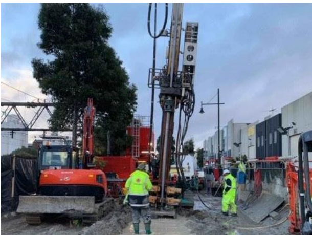
Figure 8: Jet grouting operation along rail line at CP02
