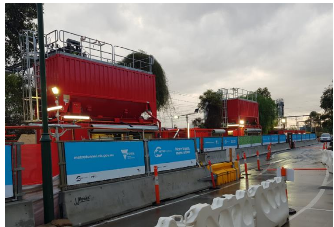
Figure 9: Batching plant set up at CP02
