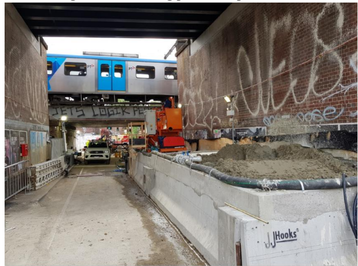
Figure 11: Spoil bay area at CP03
