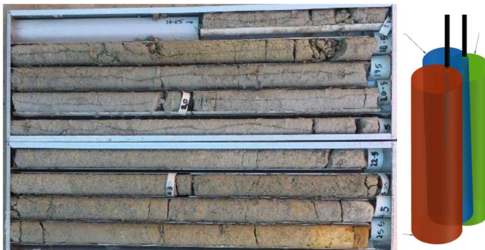
Figure 13: Cross Passage CP03 - Field trial panel D – vertical cored borehole at the triple points of columns
