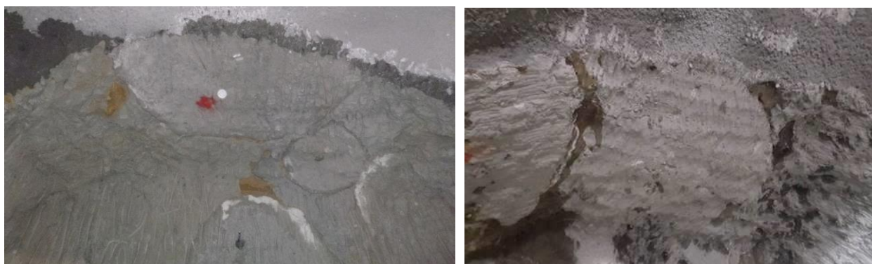
(a) Exposed JG column at CP03 (CH5.8 at mid-crown)
