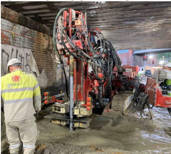
Figure 10: Jet grouting operation under rail bridge at CP03
