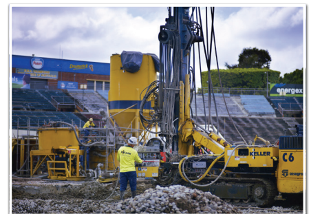
Jet Grouting over canopy of Brisbane tunnel - Keller Ground Engineering
