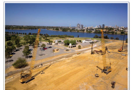
Dynamic Compaction and Wick Drains at Perth Stadium - Keller Ground Engineering
