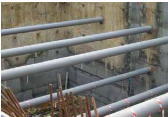
Figure 5. Steel tube struts propping east wall
