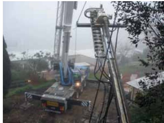
Figure 14 - Soil nail installation on the upper section of the slope
