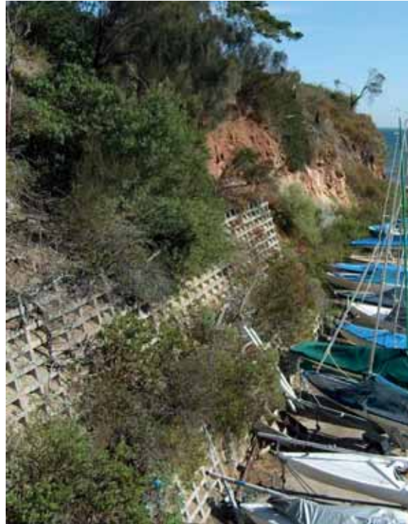
Figure 3 - Steeper area of slope including cemented zones
