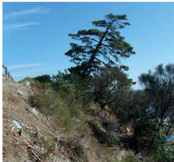
Figure 4 - Slope instability indicated by leaning trees
