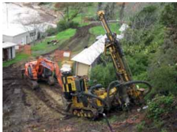
Figure 11 - Soil nail installation on the lower section of the slope
