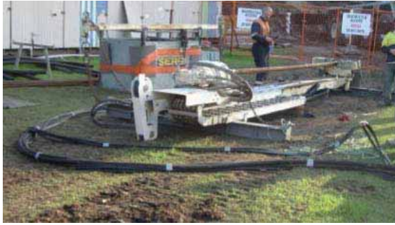
Figure 8 - The drilling rig mast with umbilical cord of hydraulic hoses attached
