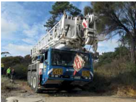
Figure 9 - The 70 tonne all terrain crane entering the site
