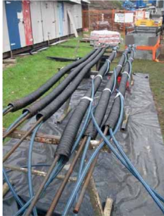
Figure 10 - Soil nail preparation on site
