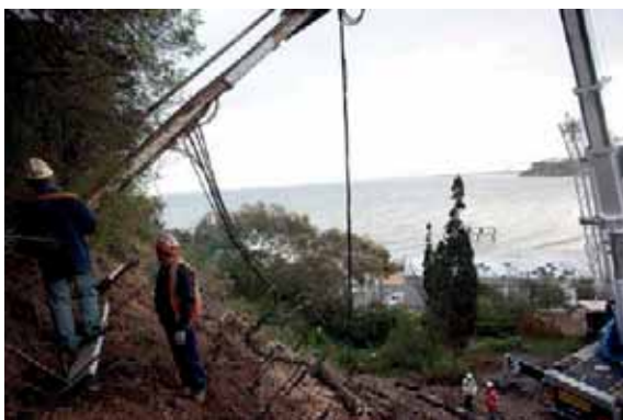
Figure 13 - Soil nail installation on the upper section of the slope
