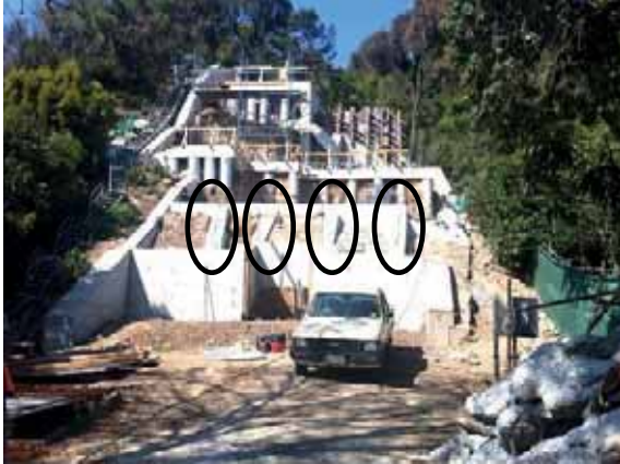
Figure 5. Foundation Arrangement (Piles & Lateral Transfer)
