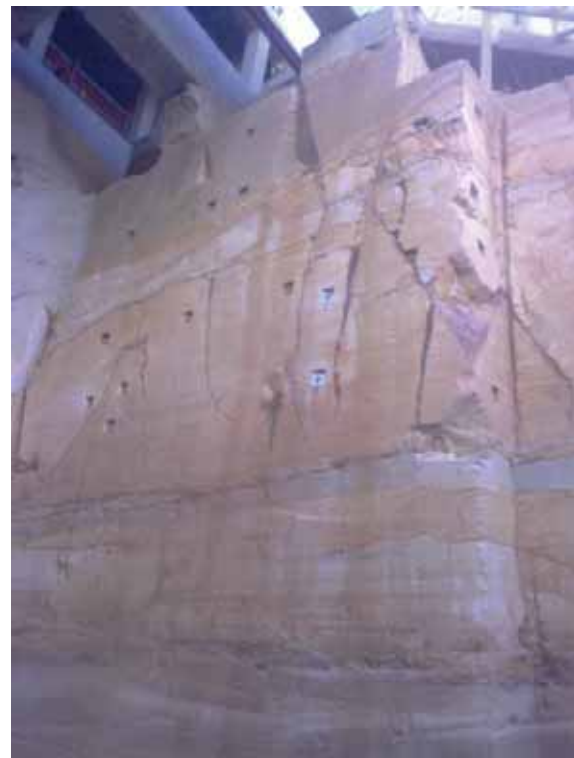
Figure 7. Example of Potential Rockfalls
