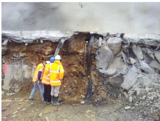
Figure 3: Highly weathered and extremely weak vesicular water carrying basalt adjacent to strong, unweathered low vesicularity basalt
