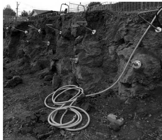
Figure 2. Example of overbreak in basalt rock
