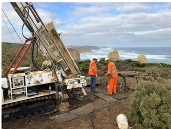
Figure 4. Inclined borehole drilling at the Saddle Lookout site
