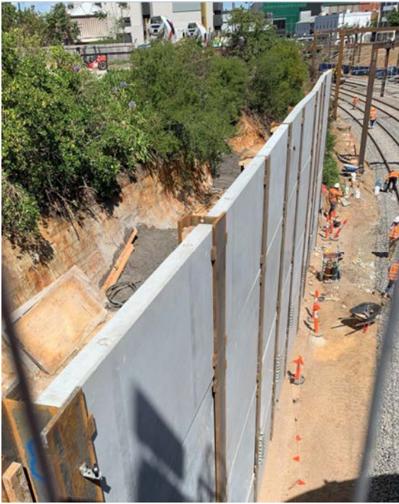
Figure 5. Backfill in progress
