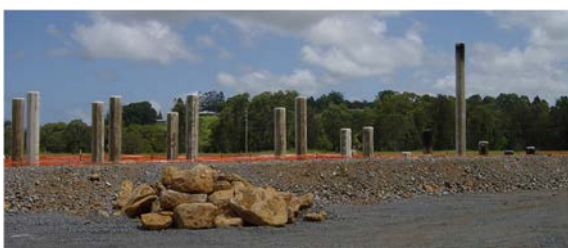
Figure 5. Piles driven onto basalt flow
