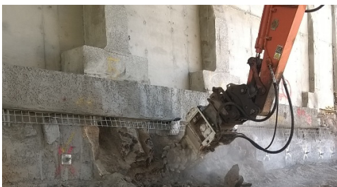
Photo 1. Rock face cutting below new continuous footing and saw cut buttresses.
