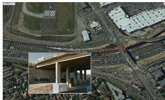
Figure 1. Bulla Road bridge north abutment location
