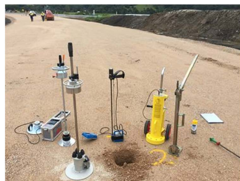
Figure 14. Various equipment used at project site
