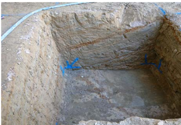
Figure 6. Spread footing with exposed HW-MW siltstone consistent with design assumptions
