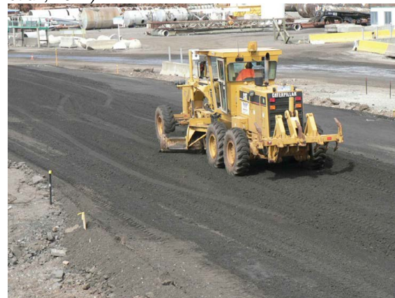
Figure 12. Construction of RG/RCA base (Arulrajah et al., 2014)
