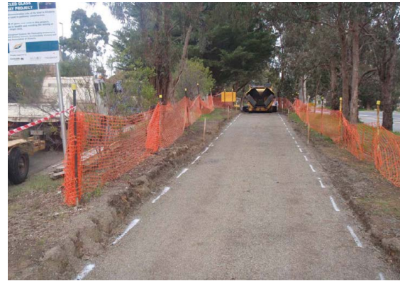
Figure 15. Footpath base sections with RG/WR blends (Arulrajah et al., 2013b)
