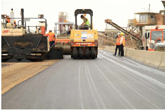
Figure 14. Construction of RAP subbase (Arulrajah et al., 2014)
