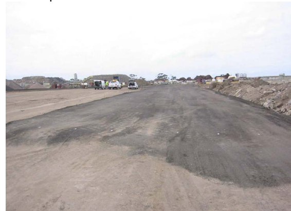
Figure 11. Construction of RAP subbase (Arulrajah et al., 2014)
