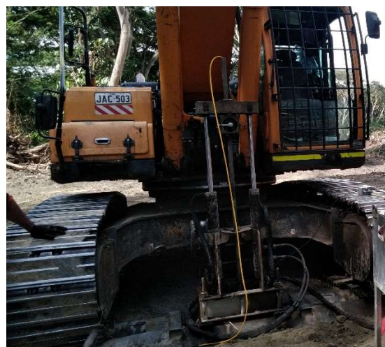
Figure 4. Portable in-situ testing rig supported by excavator
