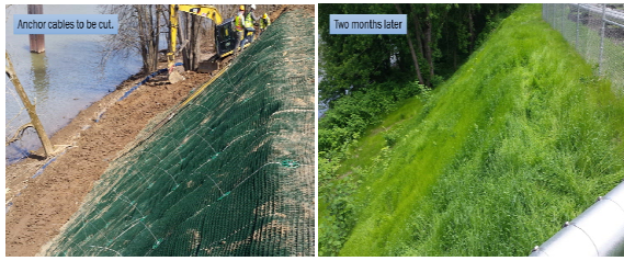
Figure 4. ARVS after installation (left) and after vegetation (right)
