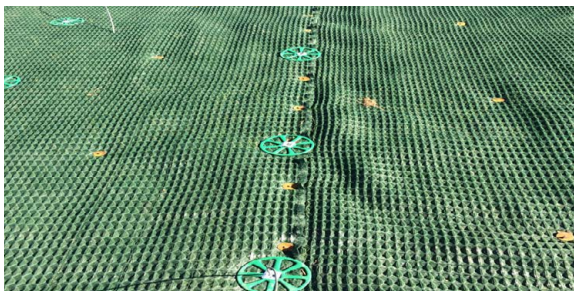
Figure 2. Homogeneous dense woven HPTRM in an ARVS
