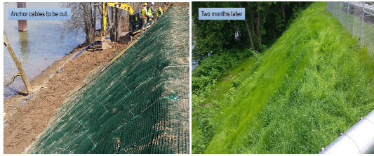
Figure 4. ARVS after installation (left) and after vegetation (right)
