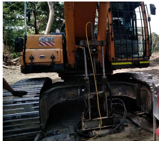
Figure 4. Portable in-situ testing rig supported by excavator
