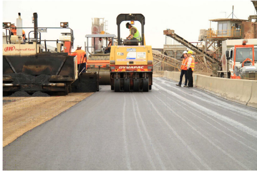
Figure 14. Construction of RAP subbase (Arulrajah et al., 2014)
