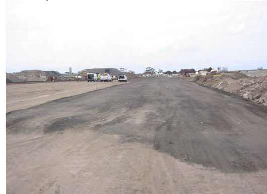
Figure 11. Construction of RAP subbase (Arulrajah et al., 2014)
