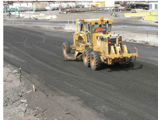
Figure 12. Construction of RG/RCA base (Arulrajah et al., 2014)
