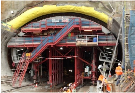
Figure 10: Undrained tunnels require greater excavations and longer construction time
