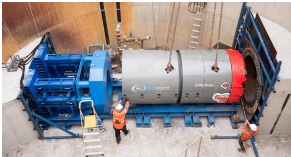
Figure 7: Microtunnel installation in caisson
