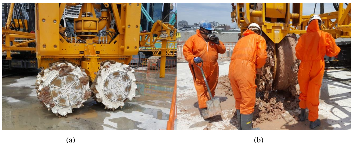
Figure 14: (a) Cutter with clean teeth; (b) cleaning cutter teeth from clayey material
