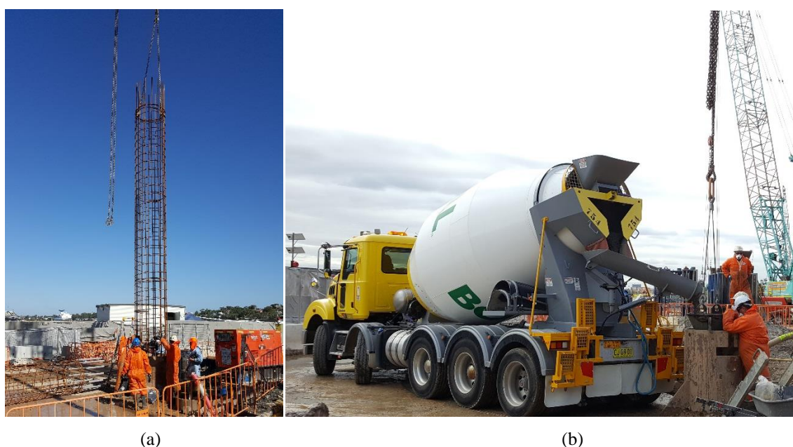
Figure 10: (a) Lowering steel cage into bentonite slurry, (b) pouring concrete
