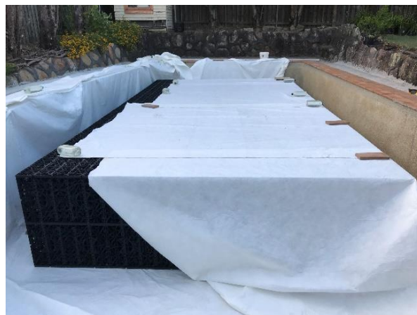
Figure 10: Double units and geofabric wrap
