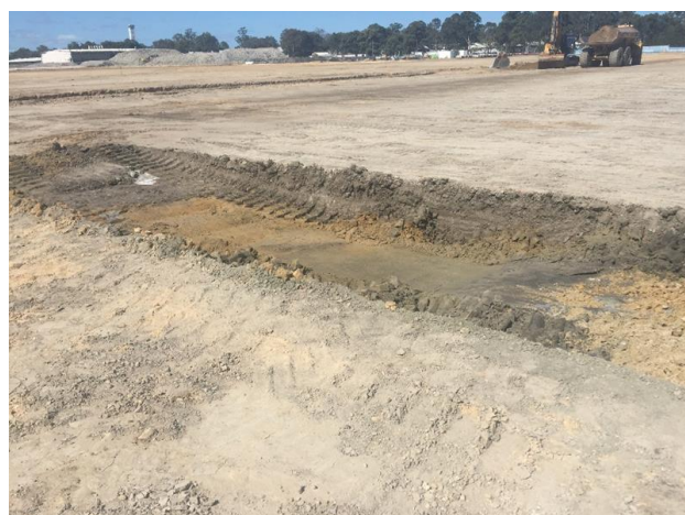
Figure 4: Removal and replace of areas post proof rolling
