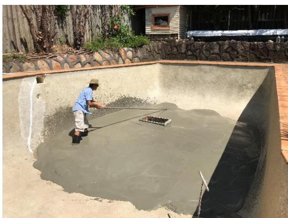
Figure 9: Placement of liquifill levelling layer
