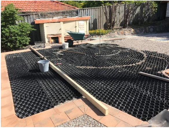
Figure 13: 40 mm thick geocell finishing layer
