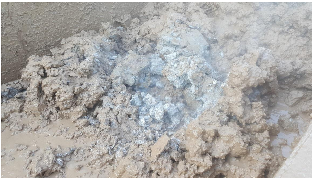
Figure 15: Excavated rock with high temperature and water vapour
