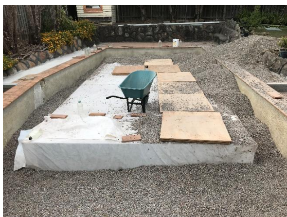
Figure 11: Backfilling around double units
