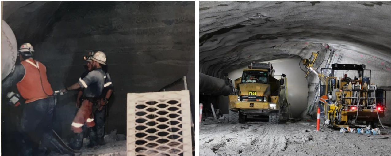
Figure 4: Hand-installed (left) and remote bolting (right)
