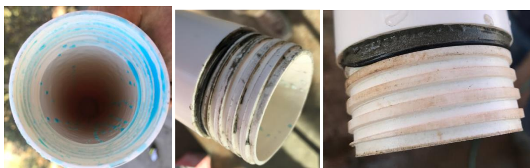
Figure 5: M/F thread with O-ring: Water breach (Left); Grout breach (Middle, Right)
