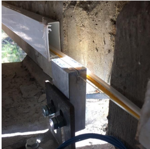
Figure 5: Longitudinal Sensor Cable Ducting
