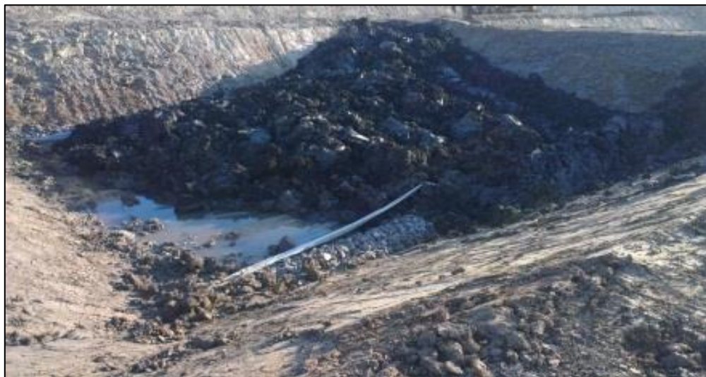
Photo 3: ASSS material midway through being dumped within trial cell by trucks.
