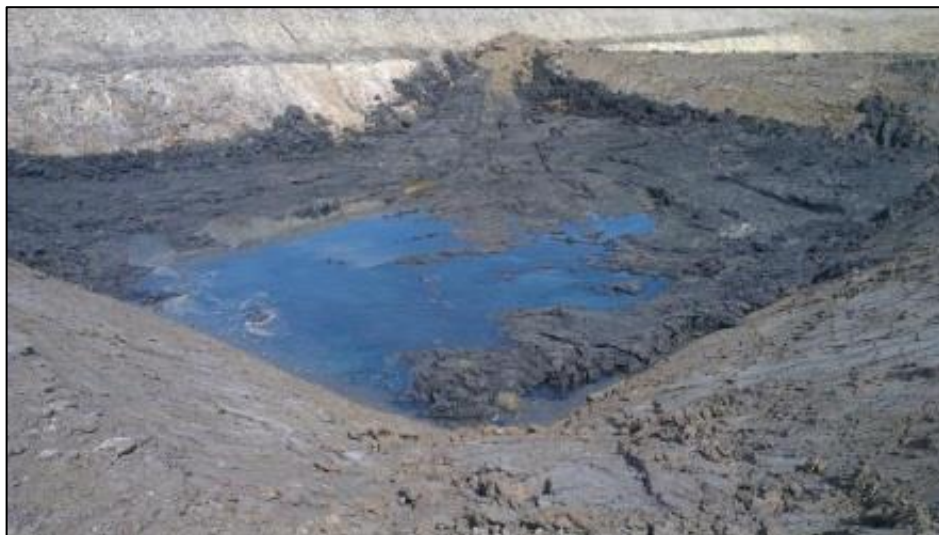
Photo 13(b): Cell T1 filled partially with groundwater that rose from the floor of the cell during a period on 10 September 2013 when pump was not functioning.
