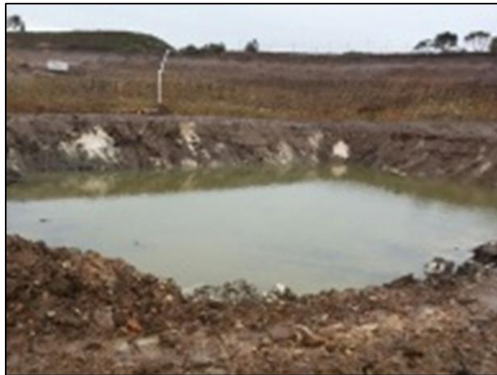
Photo 15: Rain water that filled cell T1 after placing the first layer of Hydrated lime-treated ASSS material
