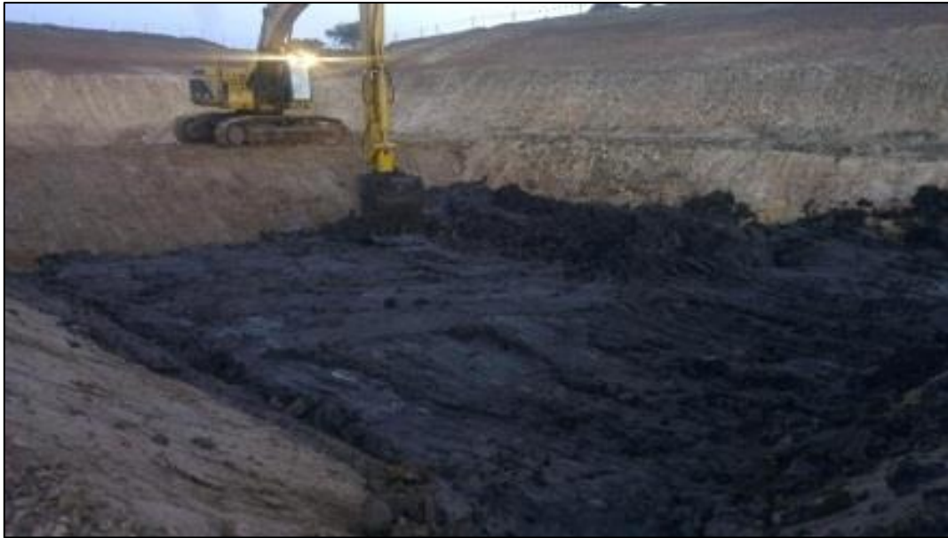
Photo 6: First layer of untreated ASSS material placed within cell T1
