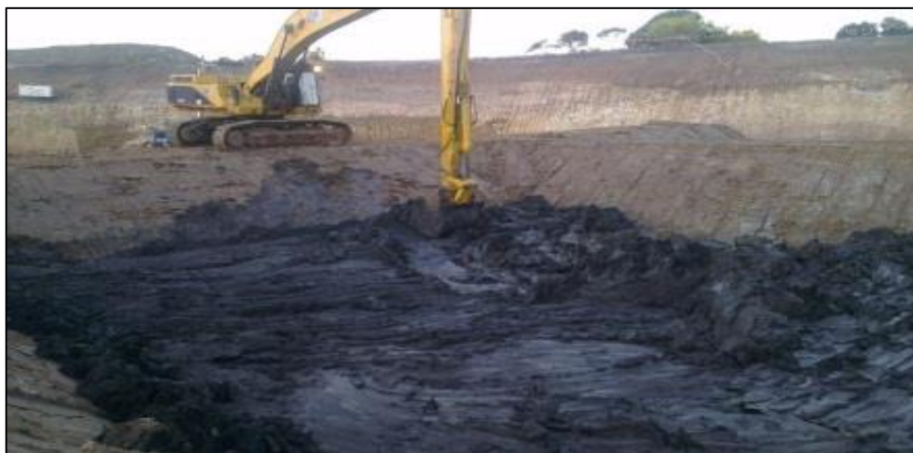
Photo 4: Long reach excavator spreading and compacting soils within trial cell T1.
