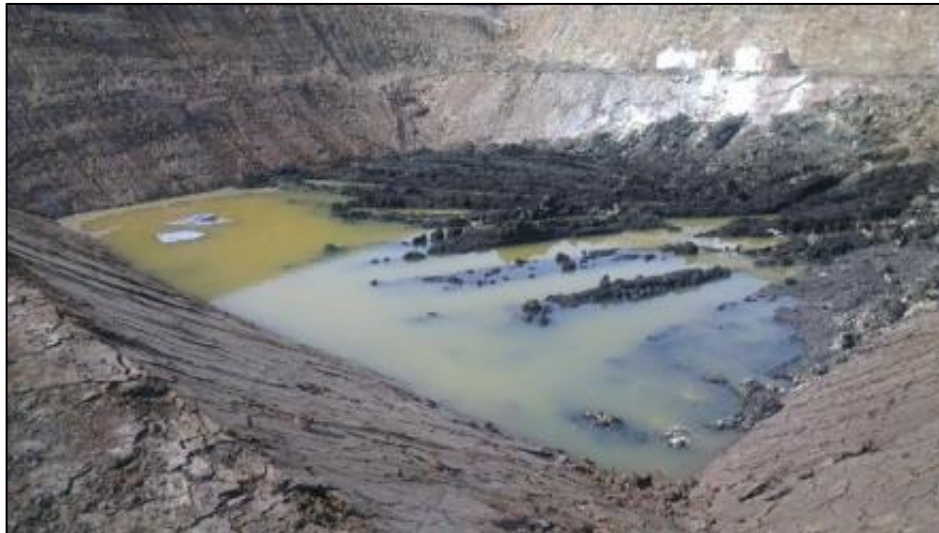
Photo 13(a): Cell T2 filled partially with groundwater that rose from the floor of the cell during a period on 10 September 2013 when pump was not functioning.
