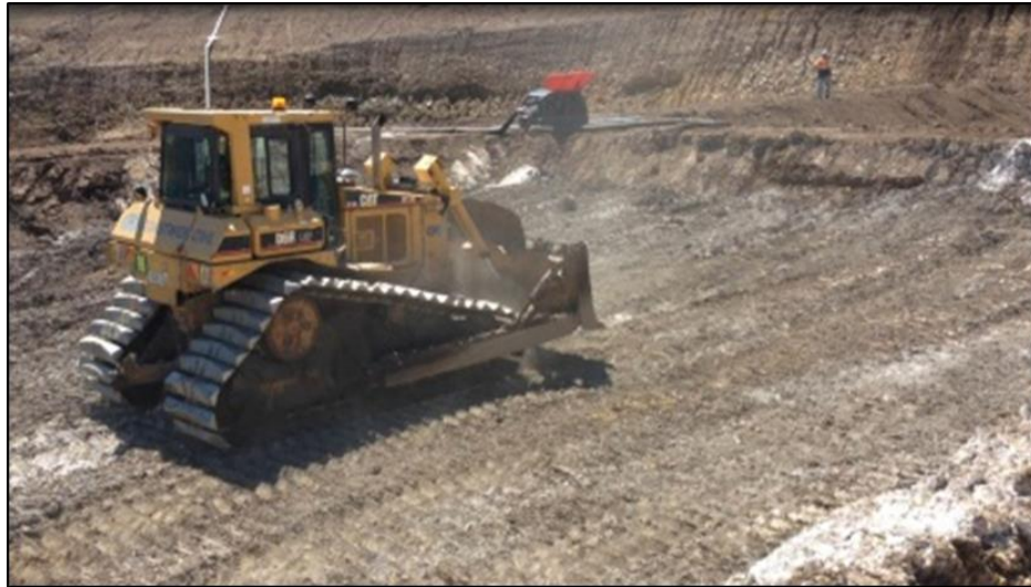
Photo 18: Swampy dozer successfully travelling on top of the second layer placed within cell T1 (treated by Hydrated lime), 12 days after placement. Note compared to Photo 17, soil surface is tight and strong.
