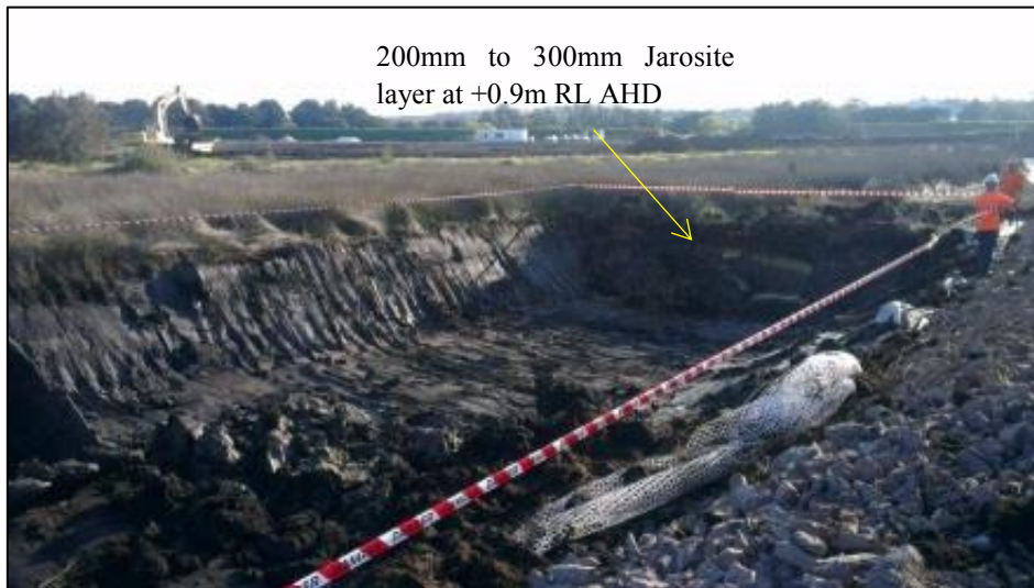
Photo 2: Extent of excavation for borrowing pit B1 and location of Jarosite layer.
