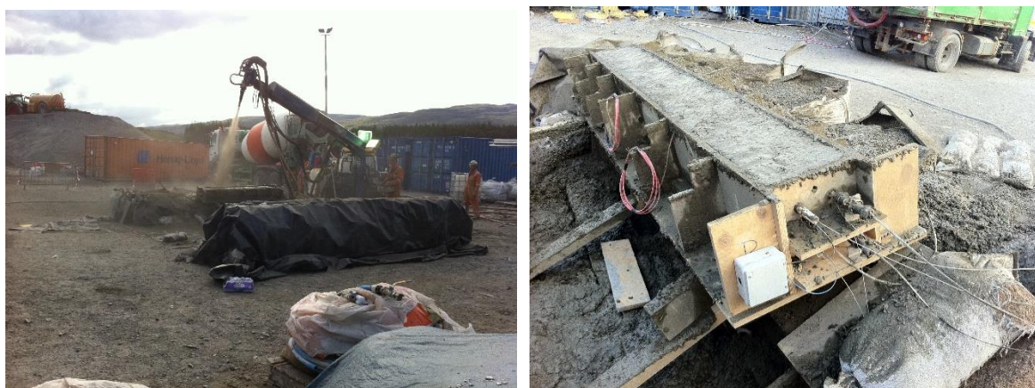
Figure 3: Sprayed Concrete Applied to Beam
