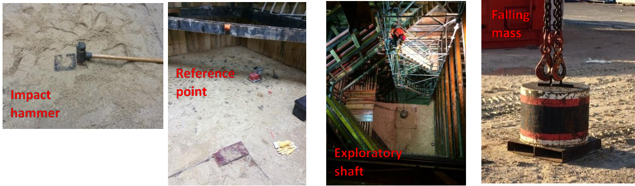
Figure 1: Installation of reference points
