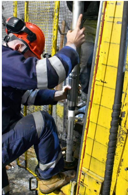
Figure 2: ANZI strain cell, data logger and installation assembly being readied for deployment in an inclined hole drilled to a depth of 740m. The collar of the hole is approximately 1340m below the ground surface.
