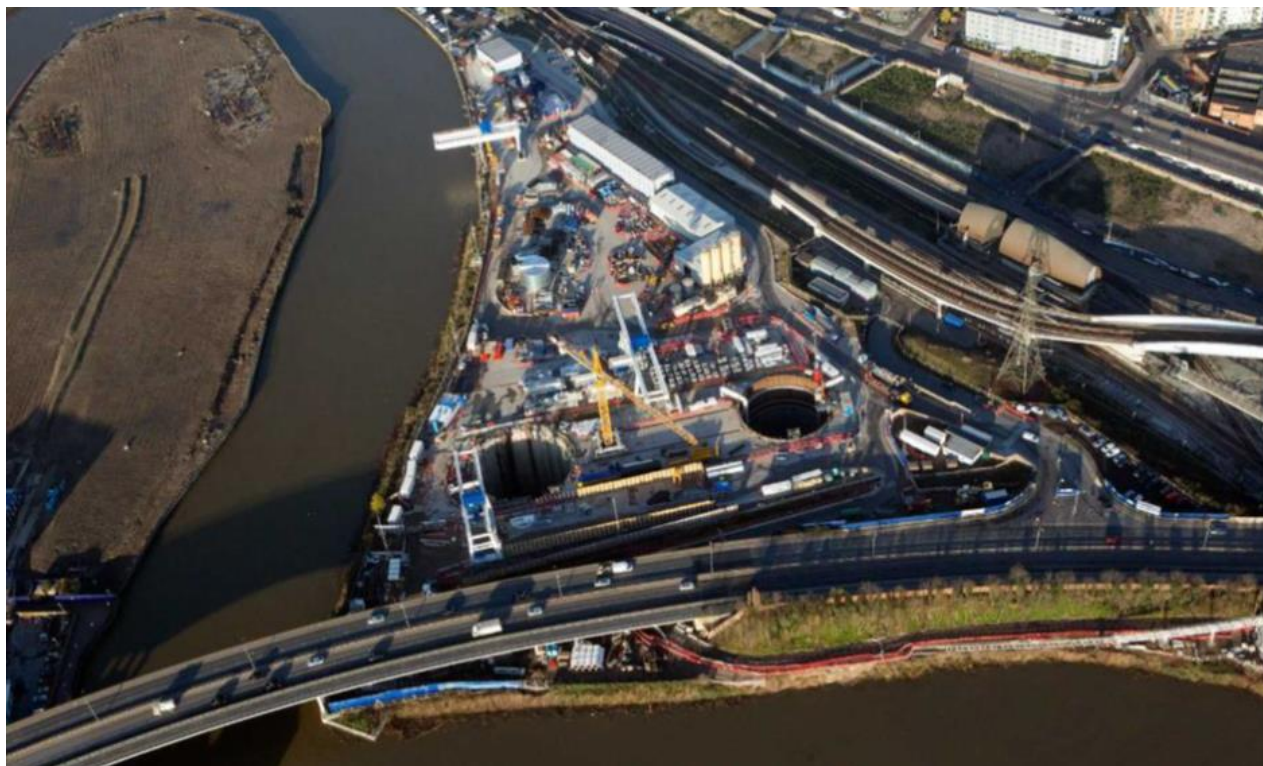
Figure 3: Limmo area while construction activity was taking place
