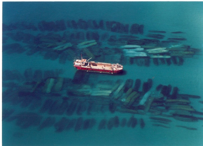
Figure 4: Placement of containers using a split hulled barge
