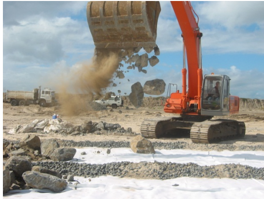
Figure 7: Trial panel set up with 3 m drop in progress.
