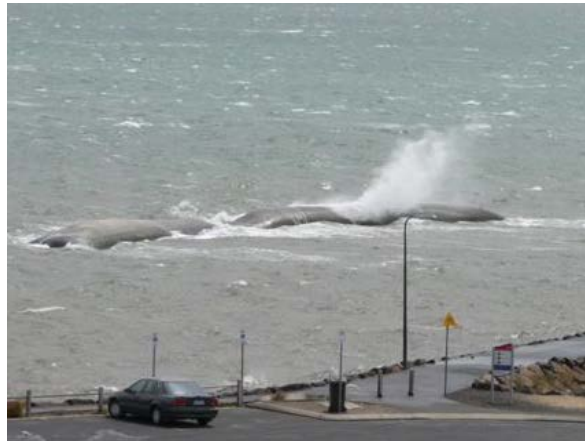
Figure 15: Limeburner's Breakwater under wave attack
