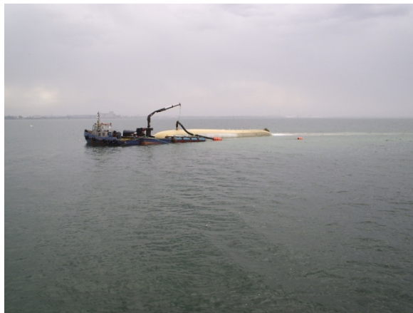
Figure 14: Geotextile tube filling
