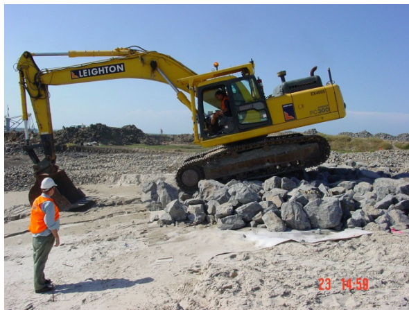
Figure 8: Trafficking with excavator.
