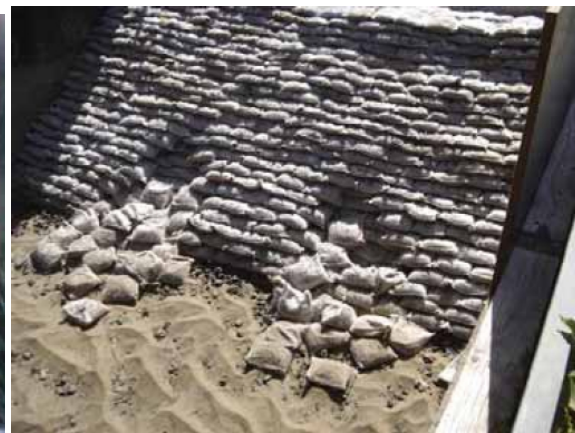
Figure 6. After wave attack (~ 15% damage)
