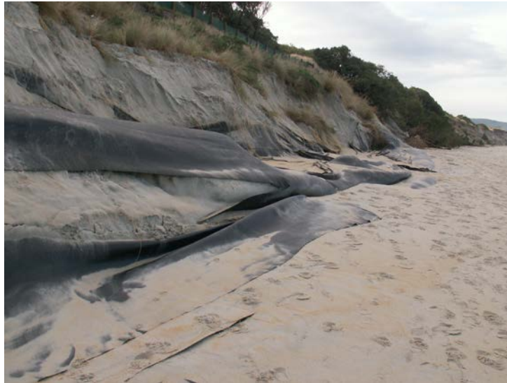
Figure 9: Vandalised geotextile tubes – St Clair Beach, New Zealand
