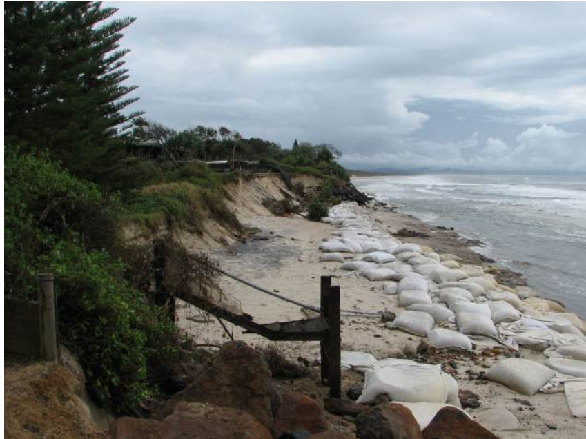
Figure 1: Sand-filled geotextile bags located seaward of eroded sand slope.
