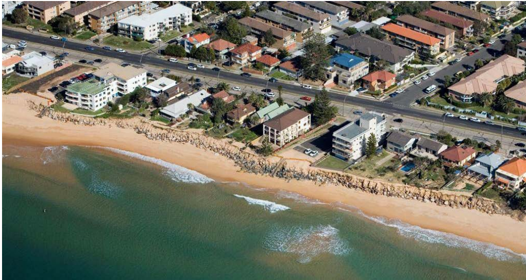
Figure 4: Historical protective works exposed at Collaroy-Narrabeen Beach in July 2007 (aerial view)
