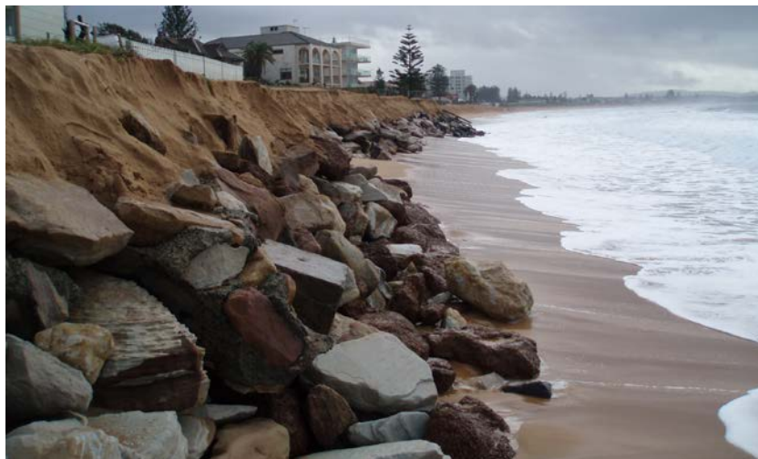
Figure 3: Historical protective works exposed at Collaroy-Narrabeen Beach in June 2007 (ground view)
