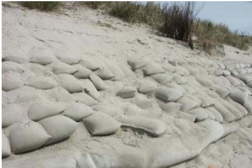
Figure 8: Sandbag pull-out on a steep dune revetment (Oumeraci & Recio 2010)
