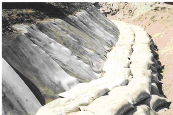
Figure 3: Left: Stockton Surf Club sand bag revetment under construction Right: Typical geotextile sand bag revetment cross-section (source Geofabrics Australasia ELCO Solutions)
