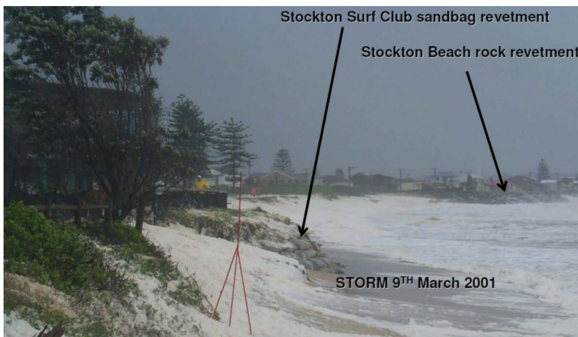
Figure 1: Rock and sandbag revetments on Stockton Beach, NSW
