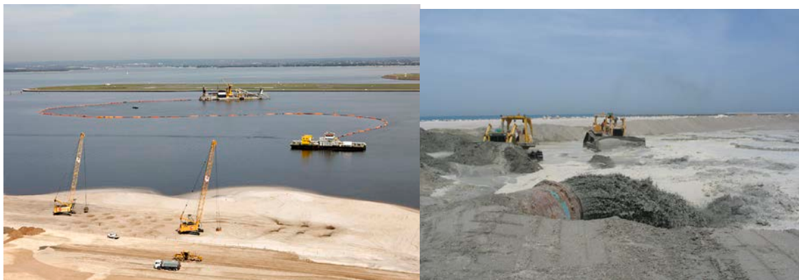
Figure 9: Reclamation activities and discharge lines
