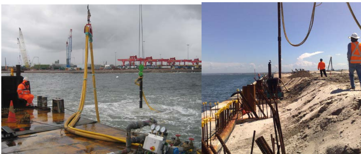
Figure 12: Marine VC (left) and near-wall VC (right)
