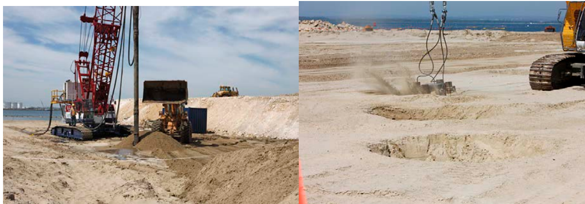
Figure 10: Land Vibrocompaction (left) and Dynamic Compaction (right)
