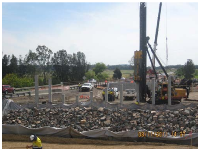
Figure 3: Piles installed at BW018
