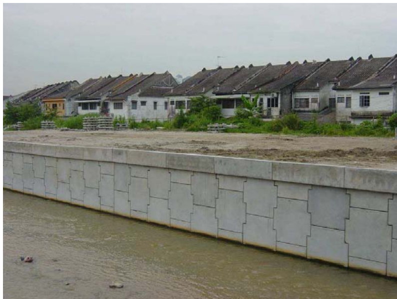
Figure 11: Marine MSE wall (GeoMega® connection system).
