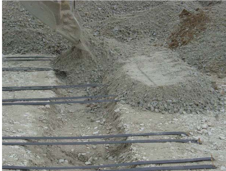
Figure 10: Backfilling operations (trench section).
