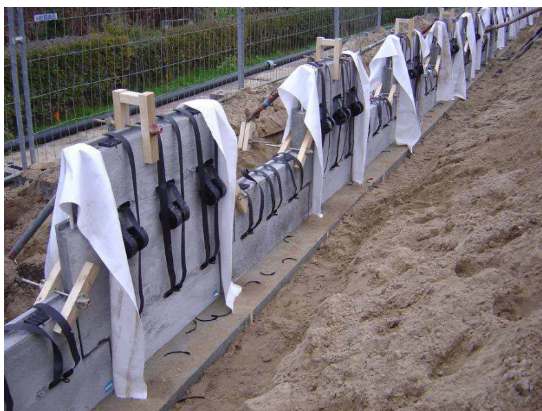
Figure 9: Initial course of facing panels set up.
