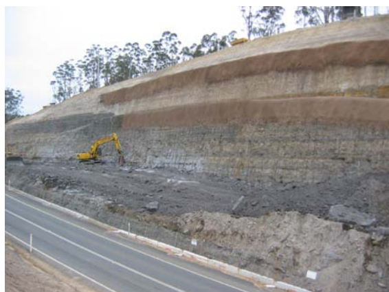
Figure 4: Cut 2 excavation of PASR - note iron oxide from oxidation of pyrite at right above first bench.
