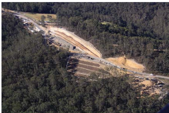
Figure 1: Conjola Mountain Fill 2, grey PASR in Cut 2.
