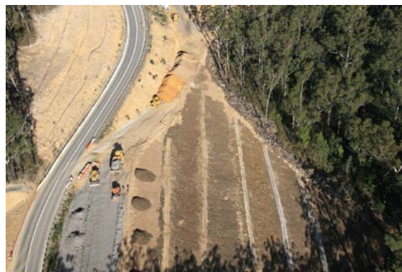
Figure 2: Fill 2 grey PASR and brown cover being placed.
