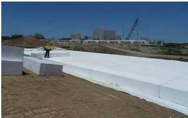
(c) Geofoam installation
