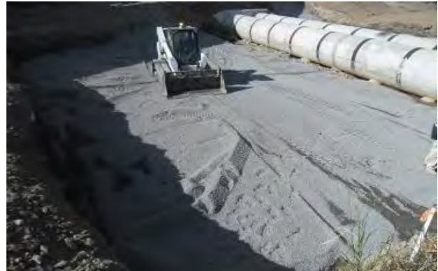
(b) Foundation preparation
