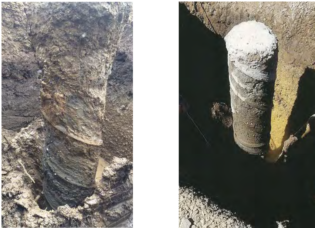
Figure 12 : Typical shape of excavated columns presenting sound characteristics
