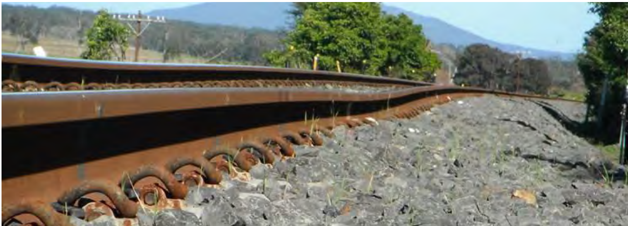
Figure 13: Track profile before retamping.
