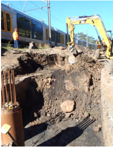
Photo 4: During construction – Proximity of construction works to existing rail line
