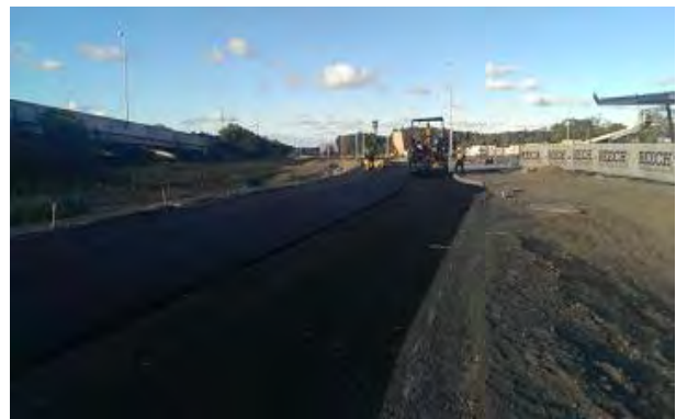
(f) Pavement construction
