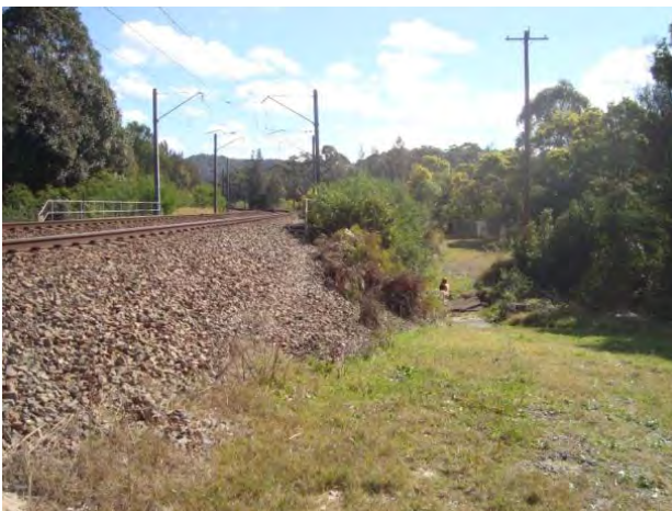
Photo 2: Pre-construction – Site of proposed rail embankment widening
