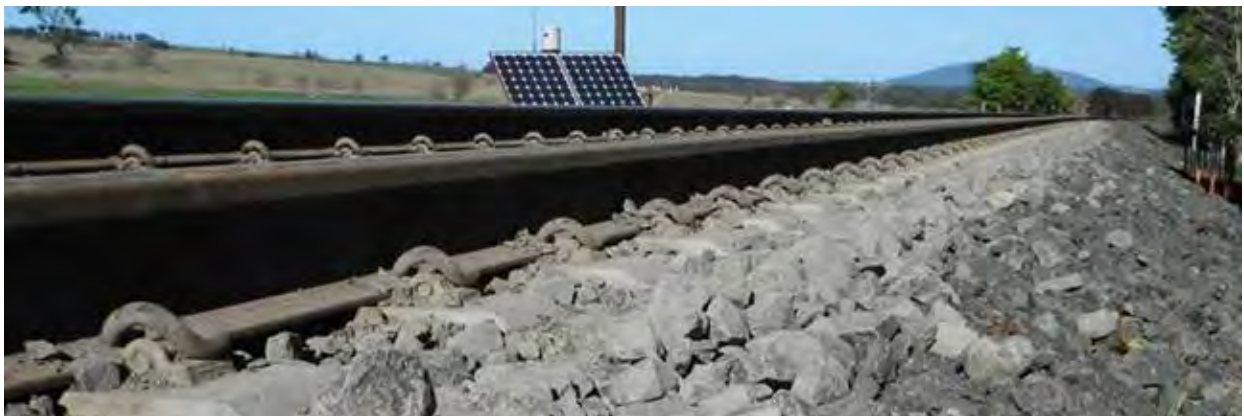
Figure 14: Track profile after retamping.
