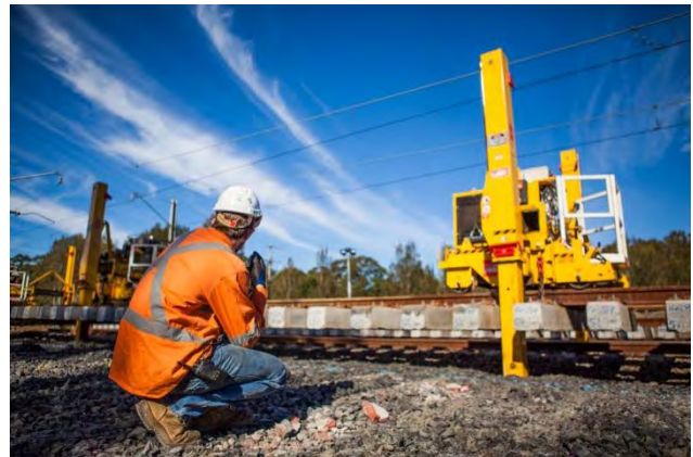
Photo 7: Construction of new rail track for Passing Loops
