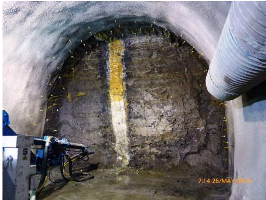
Figure 5: 800mm wide dyke in tunnel face.
