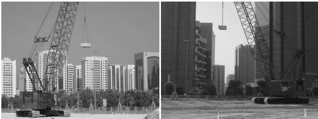
Figure 4: Dynamic compaction works in the vicinity of residential and office buildings
