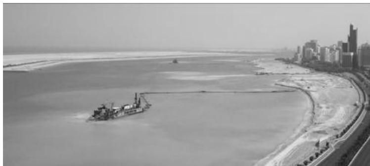
Figure 2: Pipeline hydraulic filling in Abu Dhabi Corniche
