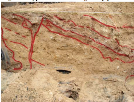
Figure 10: Section showing collapsed pipe
