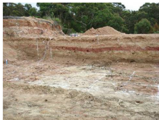
Figure 20: Dip evident in embankment fill layering
