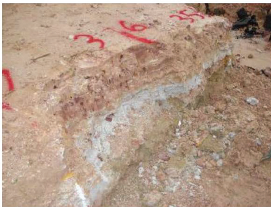
Figure 6: Trench face exposing fill layering
