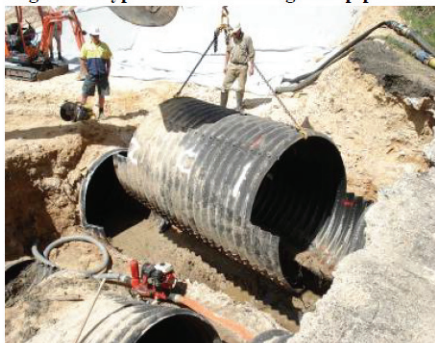
Figure 11: Pipe removal for a section of pipe
