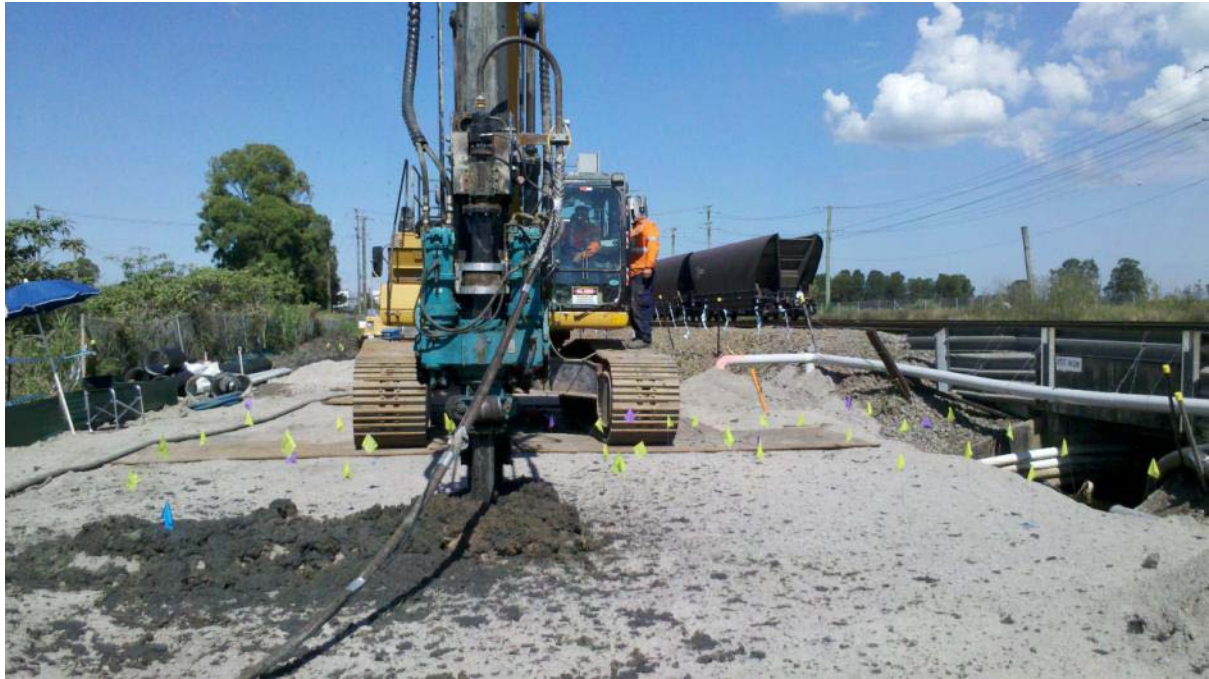
Figure 5: DSM columns construction
