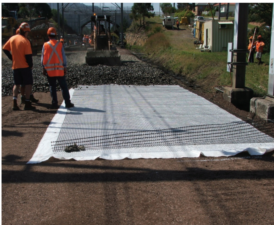
Figure 20: Installation of geocomposite under the ballast at Bulli, NSW.
