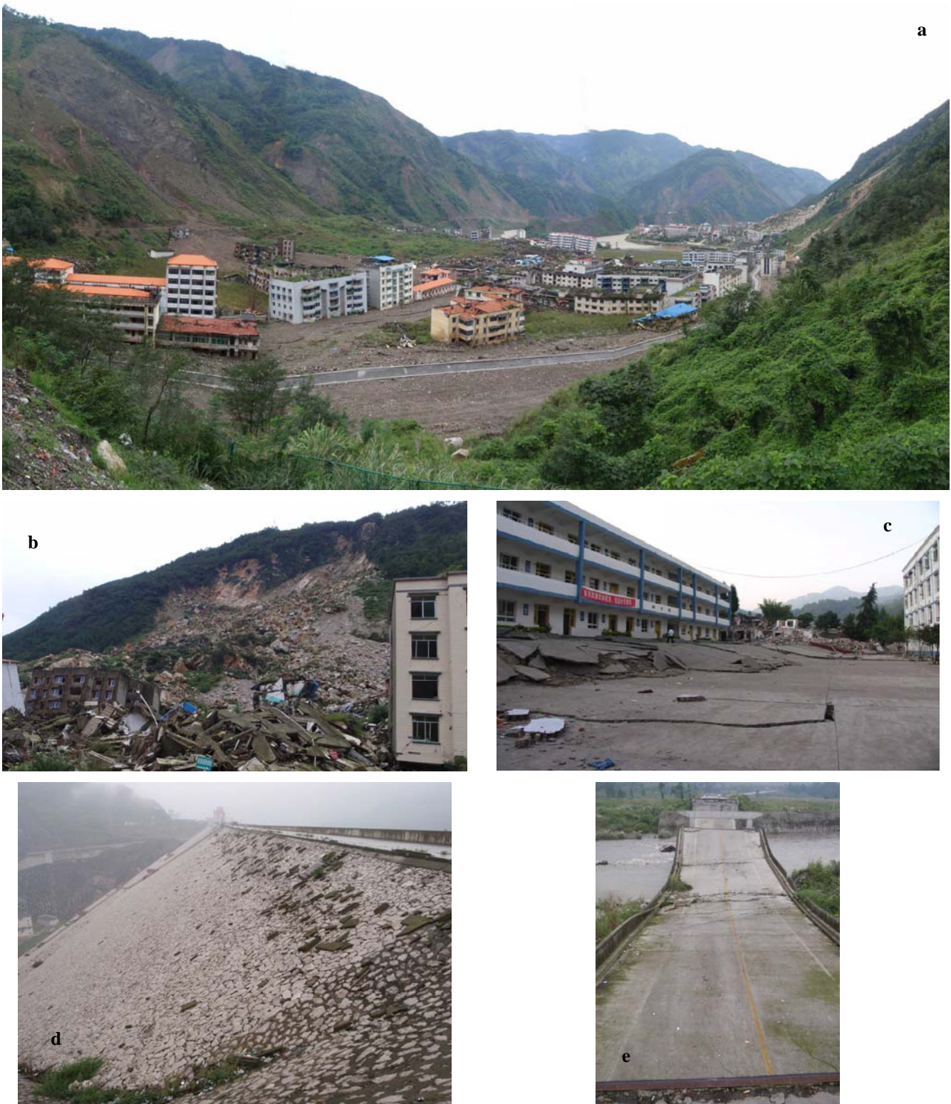
Figure 15: Examples of earthquake damage and destruction; a – overview of destruction at Beichuan Town, b – Beichuan Middle School landslide, c – fault rupture in school playground at Bailu Town, d – downstream face of Zipingpu dam, e – collapsed middle span of Xiaoyudong Bridge
