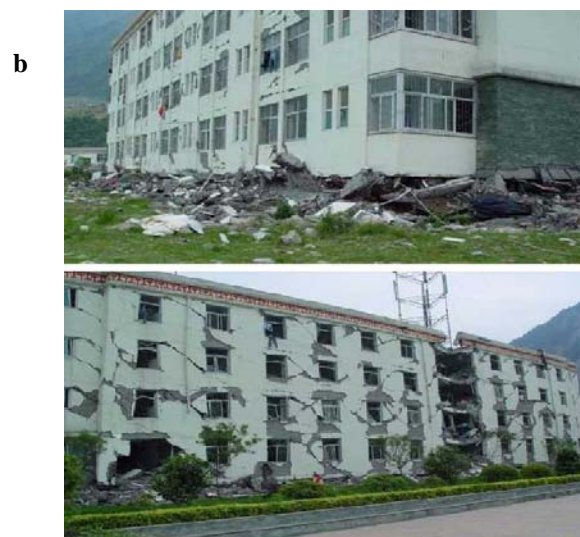
Figure 14: Examples of earthquake damage and destruction from Yingxiu Middle School; a - classroom building, b – collapsed first storey of dormitory building
