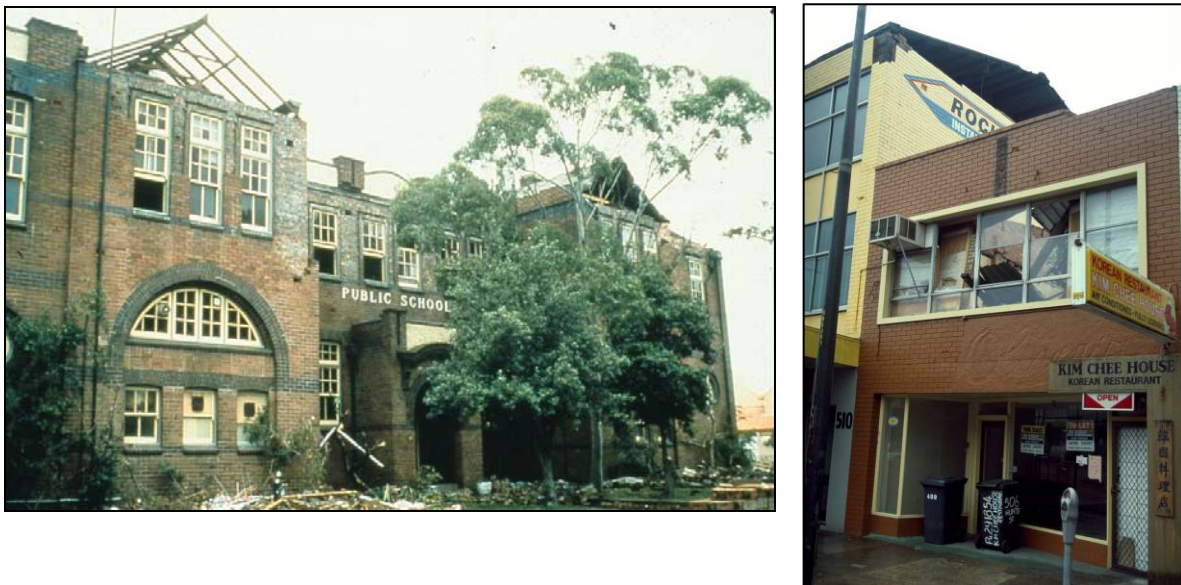
Figure 5: Examples of the more serious building damage in the Newcastle 1989 event
