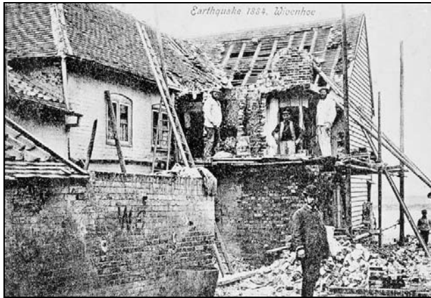
Figure 8: Example of earthquake damage in the UK
