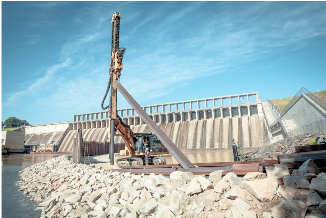
Figure 6: Sheet pile installation along earth embankment
