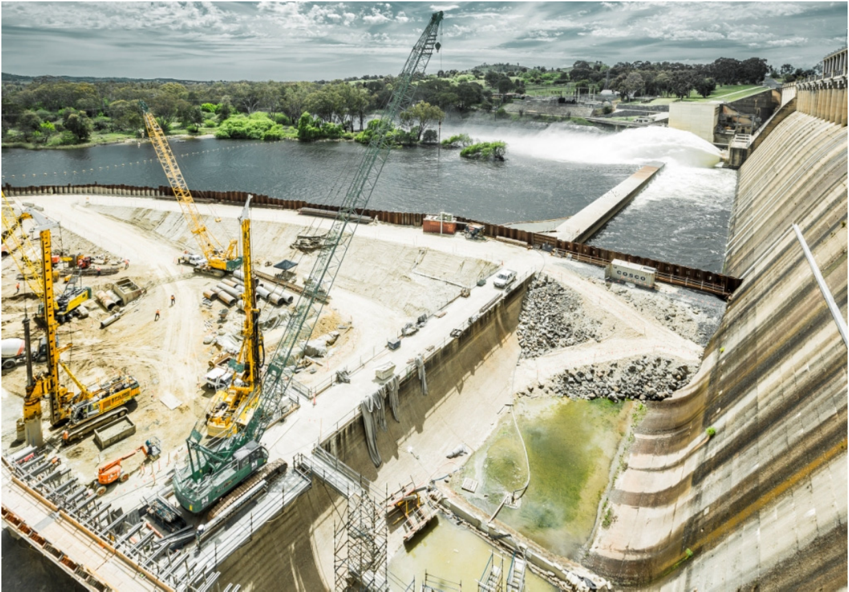
Figure 8: Pile installation within the dewatered cofferdam
