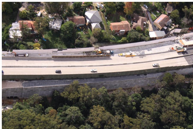
Figure 12: Aerial view of the CSRSW at its final height in June 2012.
