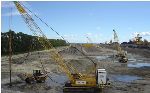
Figure 10: Top feed Vibro Stone Columns at PWCS
