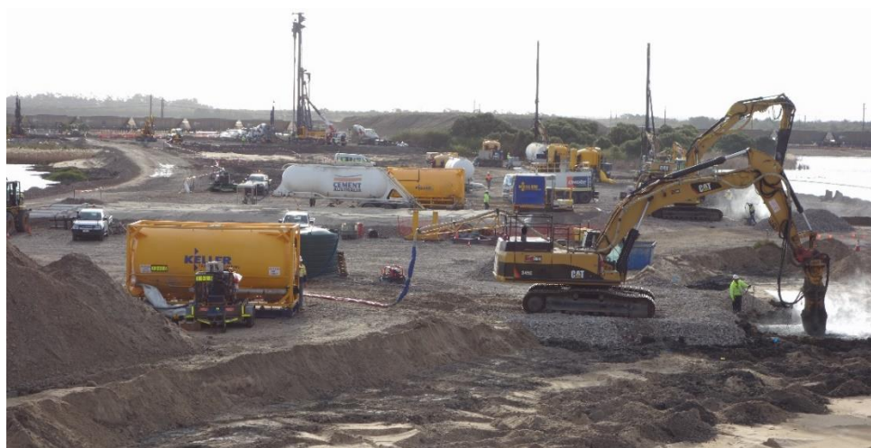
Figure 6: Simultaneous DMSM, DDSM and RI Installation
