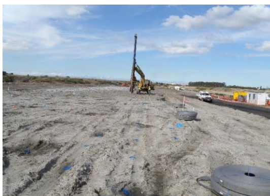
Figure 7: Installation of PVDs at PWCS CET
