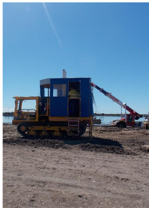
Figure 21: PORT testing of DDSM column
