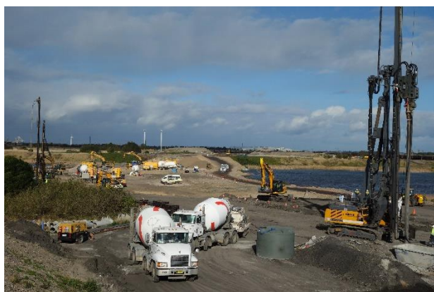
Figure 26: Concrete supply to RI rigs
