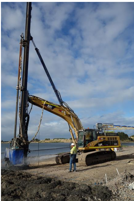
Figure 20: DDSM constructing secant column panels
