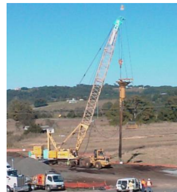
Figure 11: Bottom feed Vibro Stone Columns
