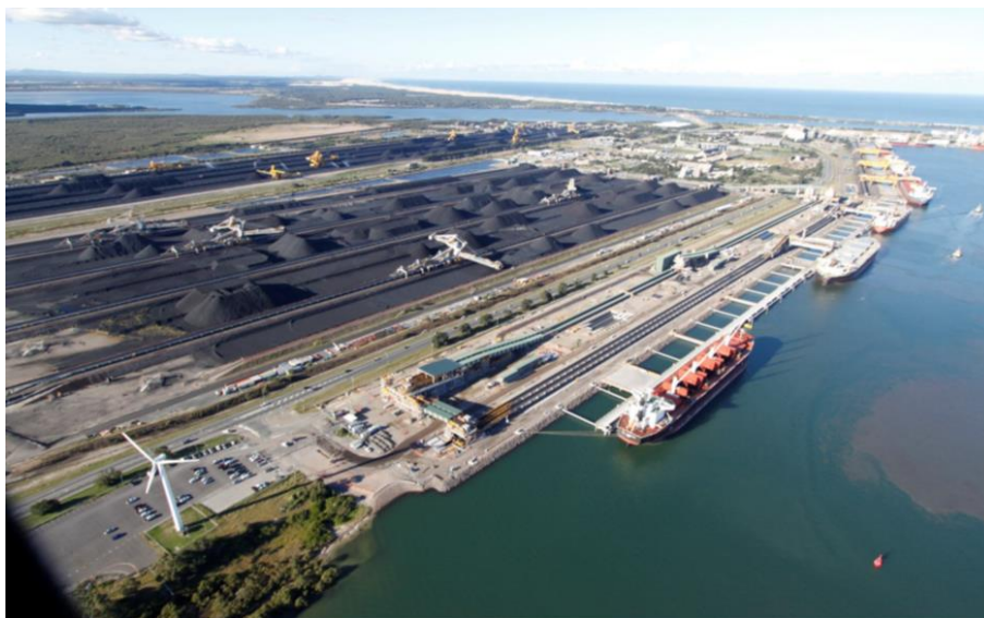
Figure 2: Coal Stockpiles, Stacker Reclaimers & Ship Loaders
