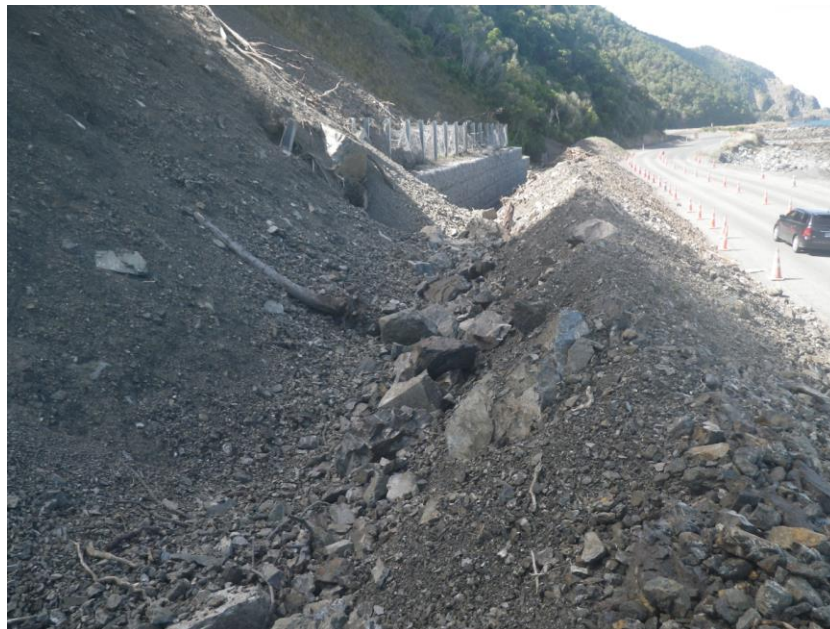
Figure 4: Temporary Rock Bunds. Note recent boulder fall.
