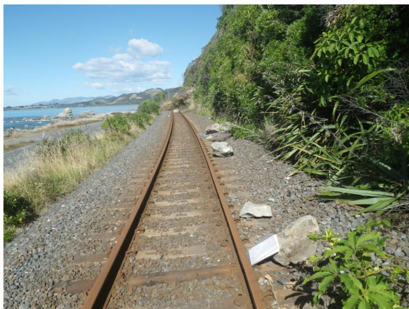
Figure 3: Railroad acting as a catch bench for rockfall
