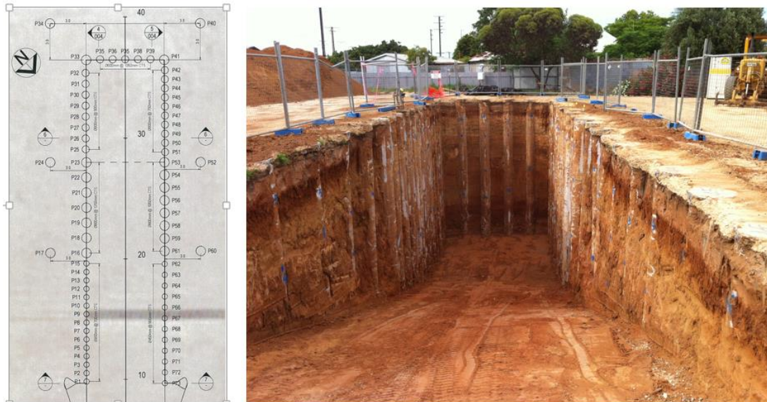
Figure 5: The trial pile wall, plan and photograph
