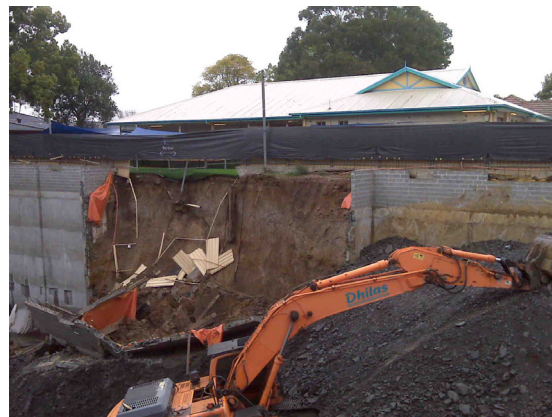
1(b) Example 2: Failure of shotcrete wall
