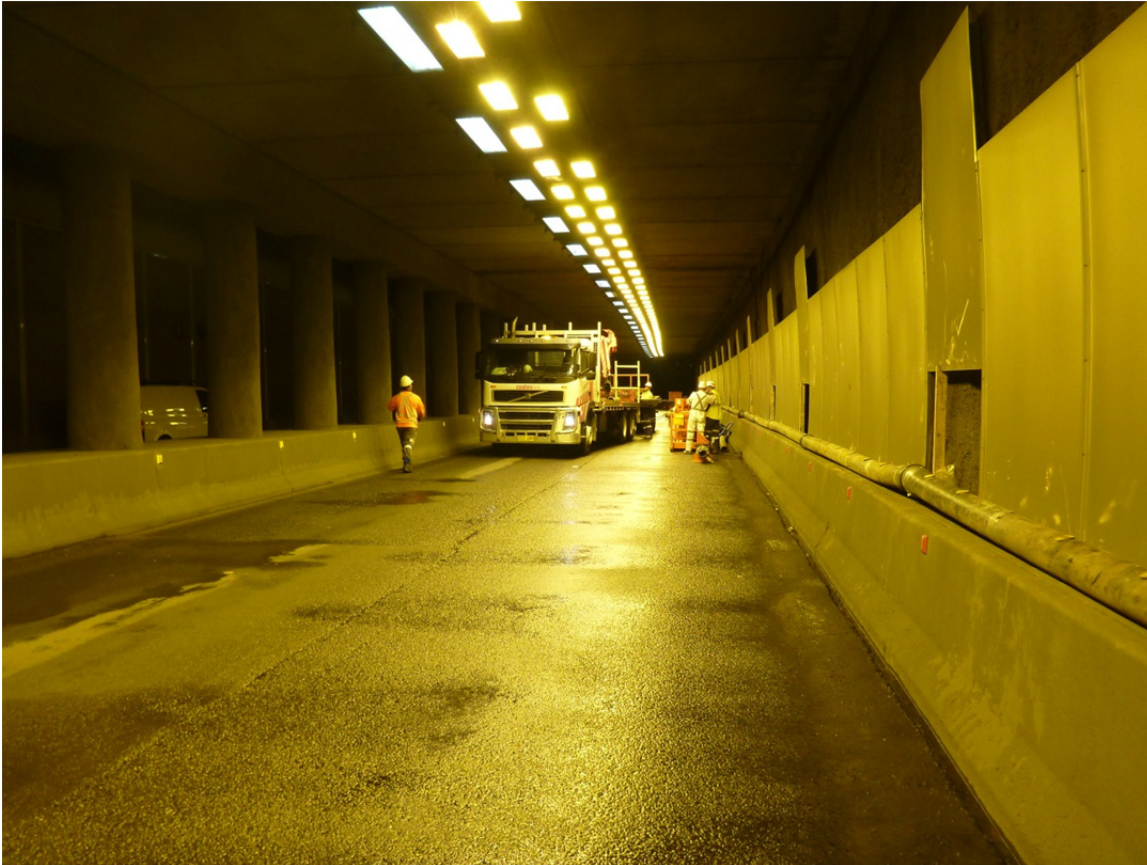
Figure 10 – Vacuum extraction manifold and relief pipe access
