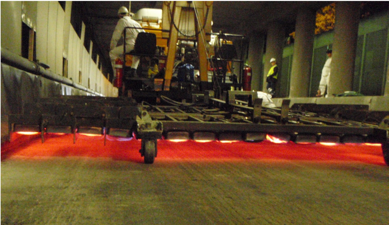
Figure 12 – Surface drying in preparation for asphalt placement
